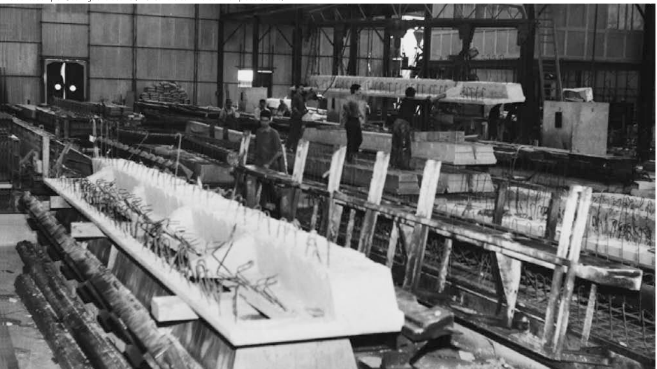
Prefabrication plant, ceilings and beams (© G. Carrard et M. Vardon/Pompidou Centre)
