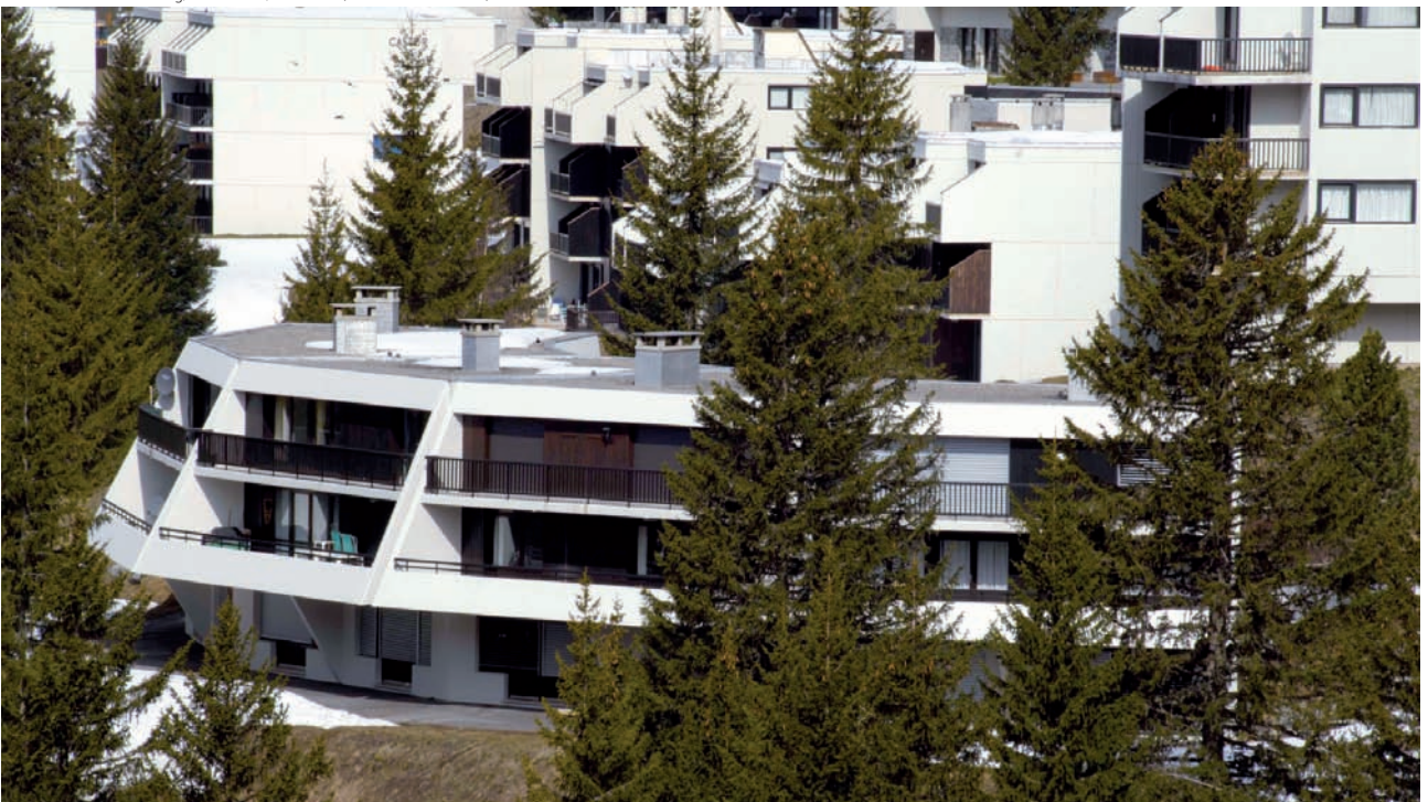
The Grands Vans building, G. Chervaz, architect (R. Bianchi/CAUE 74)
