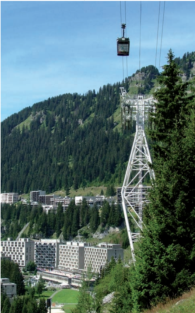
Pylon No. 1 of the Flaine cable car (G. Coquard/CCF)
