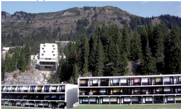
Flaine Front de Neige, general view of the facades (CAUE 74)
