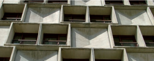
1, 2 & 3 : Les Lindars Hotel, detail of box windows and diamond pattern panels (G. Coquard/CCF)
