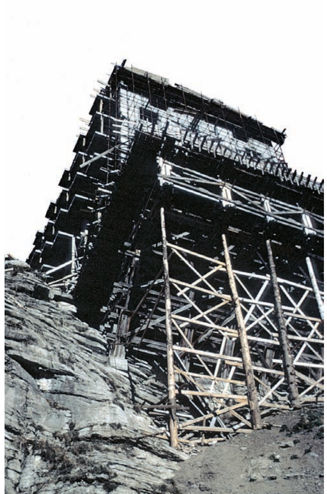
Le Flaine Hotel, cantilever scaffolding, 1967 (© Carrard G. and Mr. Vardon/ Pompidou Centre)
