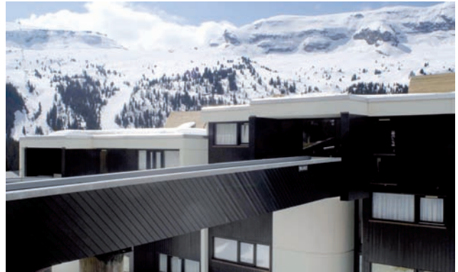
The Balance Building, walkway and cladding in painted wood (R. Bianchi/ CAUE 74)
